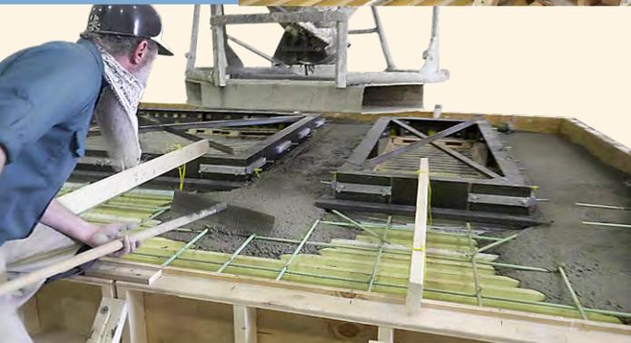
Rebar is positioned over the form and concrete is cast. A layer of insulation is sandwiched between two layers of reinforced concrete.
