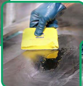
A scraper is used to level Black Panther™ 85 over the torn area .
