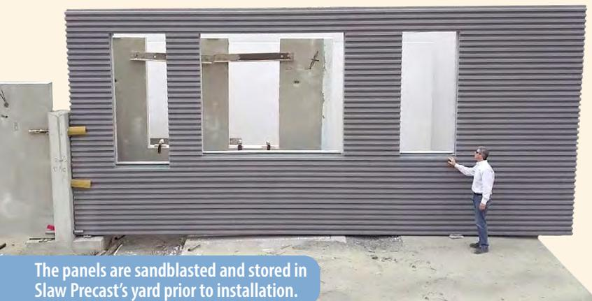
The panels are sandblasted and stored in Slaw Precast's yard prior to installation.
