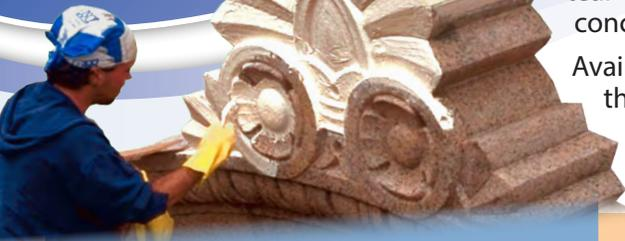
MJM Studios applied **Brush-On™ 40** on-site to create the architectural mold used to restore the arch atop New York City's landmark Bellevue Hospital.
